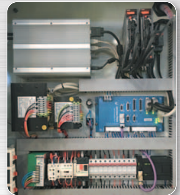
*Nexcom industrial grade fanless PC *i7 CPU/2G DDR3/128G SSD HDD
